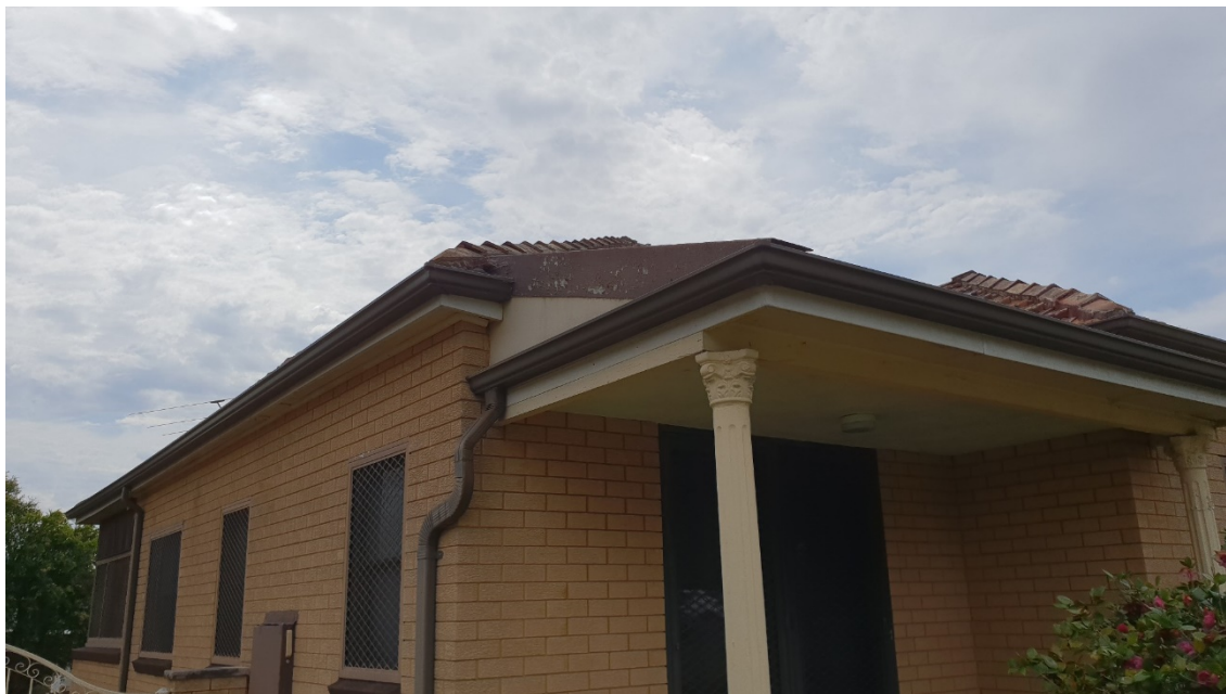
Photograph No. 4: Moulded asbestos cement capping to west side of roof over the front verandah. The small dutch gable is clad with flat asbestos cement sheet
