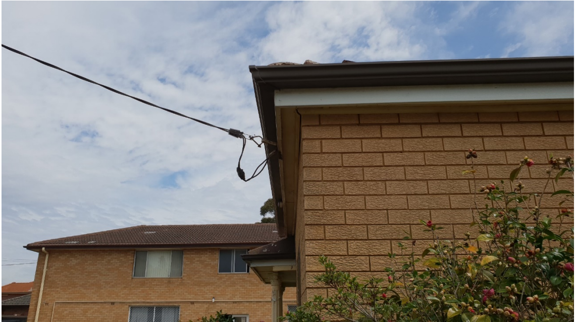
Photograph No. 5: Narrow flat asbestos cement sheet eave lining on house at 71 Kerrs Road, Lidcombe. Most of the eave lining and the asbestos cement sheet wall cladding is concealed behind the brick veneer wall cladding
