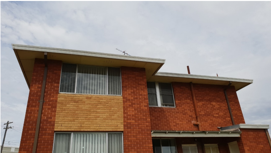
Photograph No. 2: Asbestos cement sheet eaves soffit lining on the rear of the house at 65 Kerrs Road, Lidcombe NSW
